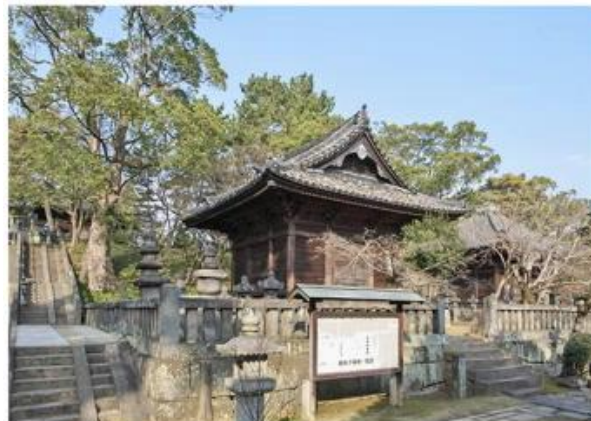
Bairin'in Ancestral Hall (foreground) and Shunrin'in Ancestral Hall (background)
