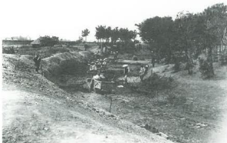
During the restoration work
